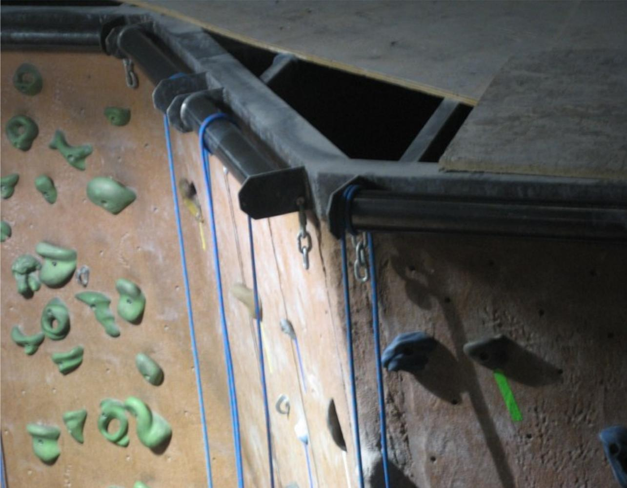
A Belay Bar is usually a 4-inch in diameter bar that is anywhere from 4 feet to 8 feet long welded securely at the top of the wall. You could also bolt it to the structure. A rope is then wrapped around the bar **TWICE** which creates a coefficient of friction for the belay.
